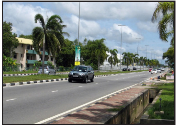
Well-built roads connecting Serusop to the other areas.
