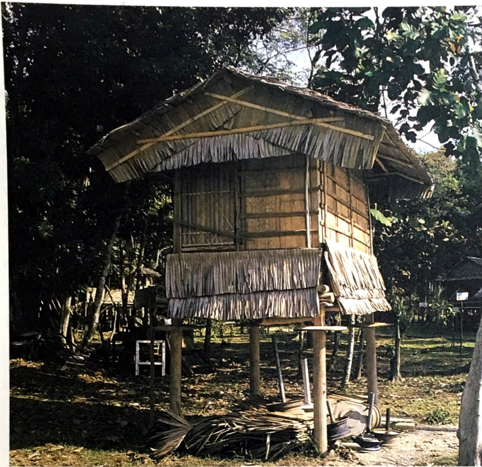
The "Durong" with thatched wall and thatched roof (thatch palm). Note the circular dinar on each of the four posts.
