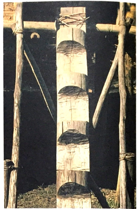
The ladder, known as "Tangga Kambing" which literally translates as "Goat ladder" is made of a single tree trunk with notches carved out at fairly even intervals for footing. It is believed that it is called the goat ladder because goats are probably the only animals that can climb on such a ladder. No doubt, this could be true with the nimble-footed mountain goats.
