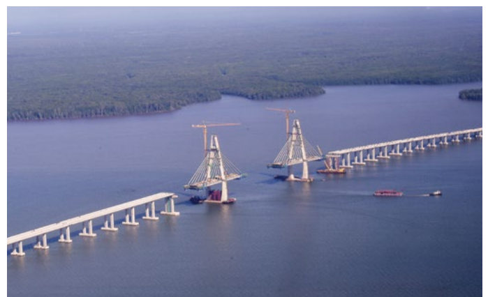
An aerial view of the construction progress of the Temburong Bridge.
