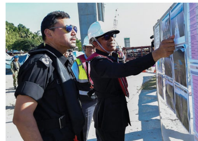
His Royal Highness being briefed by Yang Berhormat Dato Seri Setia Awang Haji Suhaimi bin Haji Gafar, Minister of Development, on the construction activities of the Temburong Bridge.
