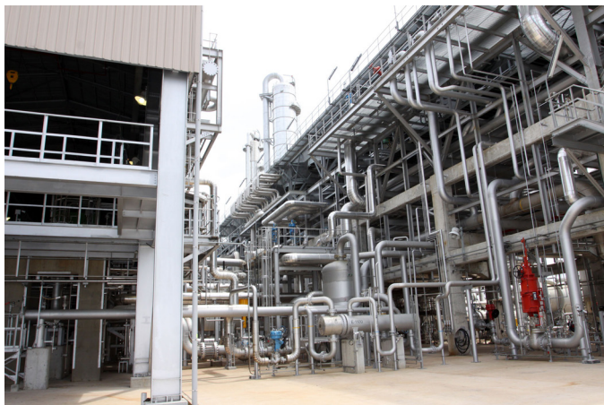
Part of the Industrial Gas Terminal (IGT) area that launch.
